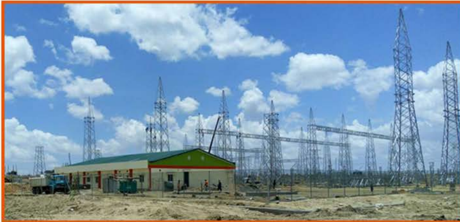
Isinya substation - staff housing
