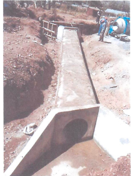
Construction of 900mm cross culvert
