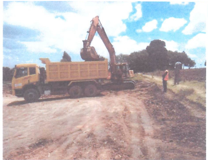
Excavation of top soil and cart away
