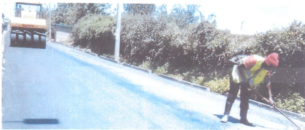
Compaction of AC using PTR Machine
