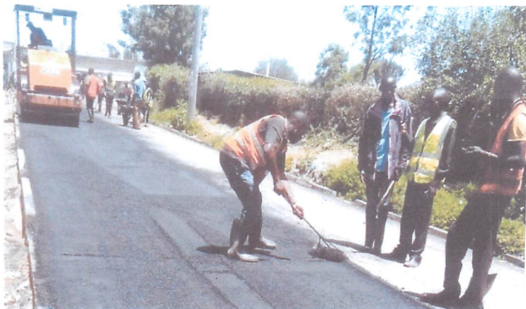
Leveling and Compaction of AC
